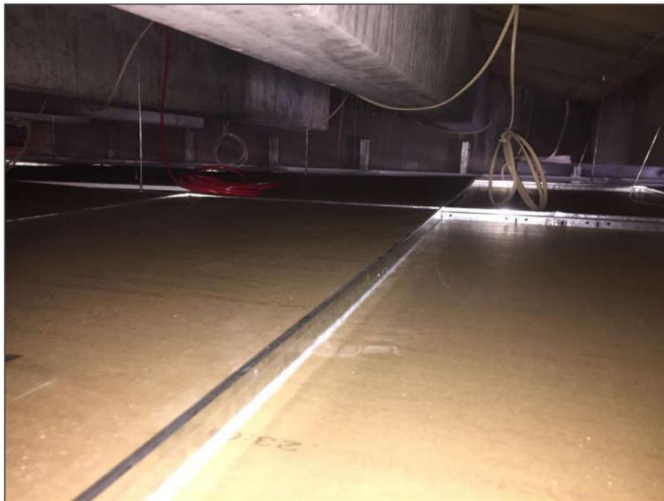
Figure 2: Ecoplus Fastlock System - Overloaded grid tiles
