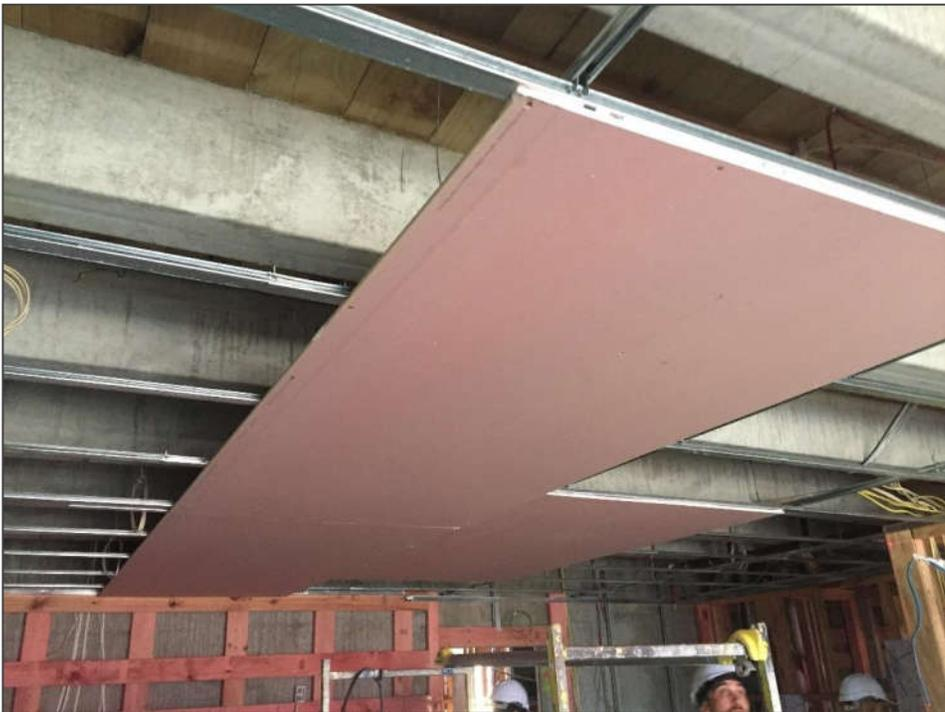
Figure 4: 16mm Plasterboard Grid System - Installed ceiling (part)
