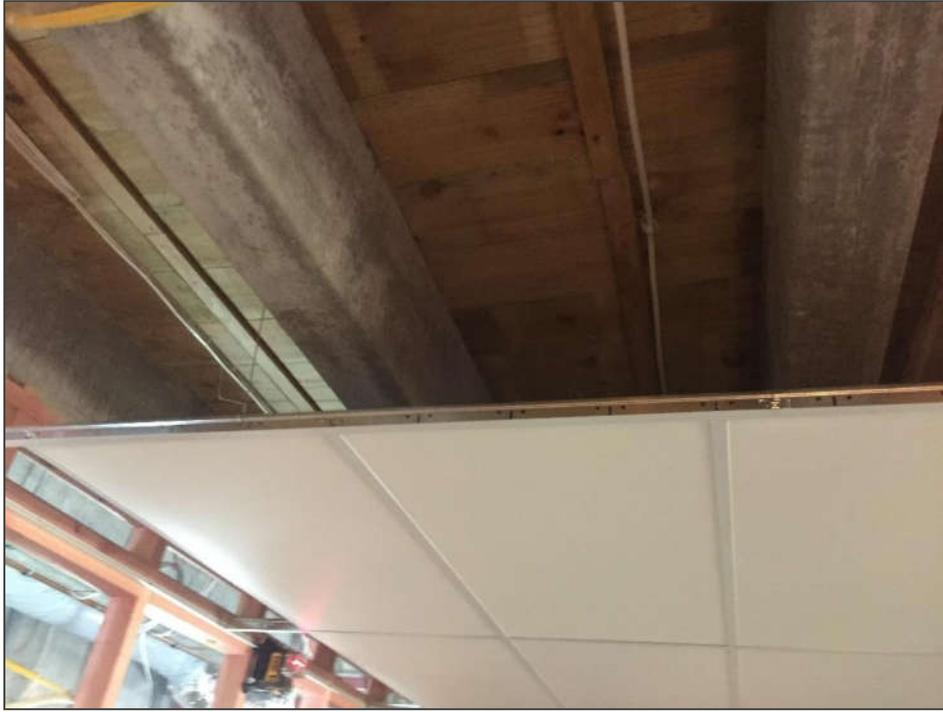
Figure 1: Ecoplus Fastlock System - Installed ceiling
