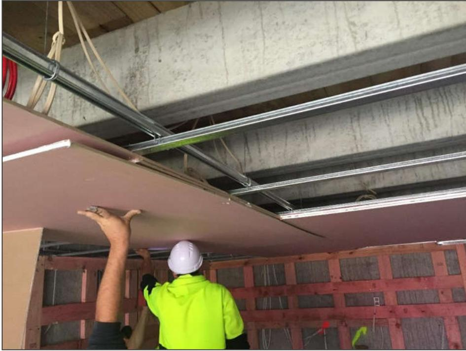
Figure 5: 16mm Plasterboard Grid System - Installation of third layer of GIB
